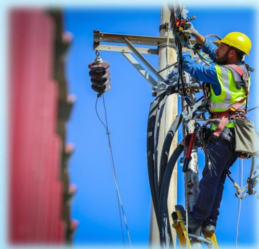
Added Low Voltage Network lengths 294.1 KM
